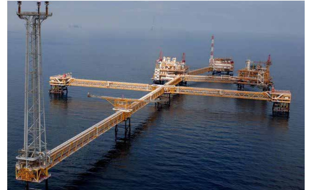
A scene of North Field, where the majority of Qatar's natural gas is located
