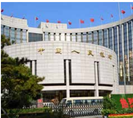
People's Bank of China headquarters in Beijing
